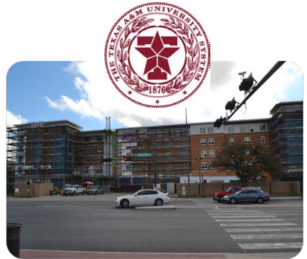
TAMU Northside Residence Hall College Station, TX
