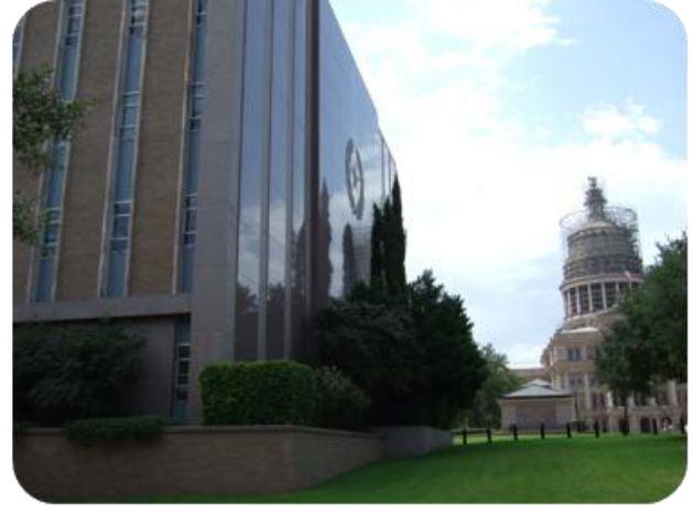
Texas Workforce Commission Cooling Tower Replacement Project Austin, TX
